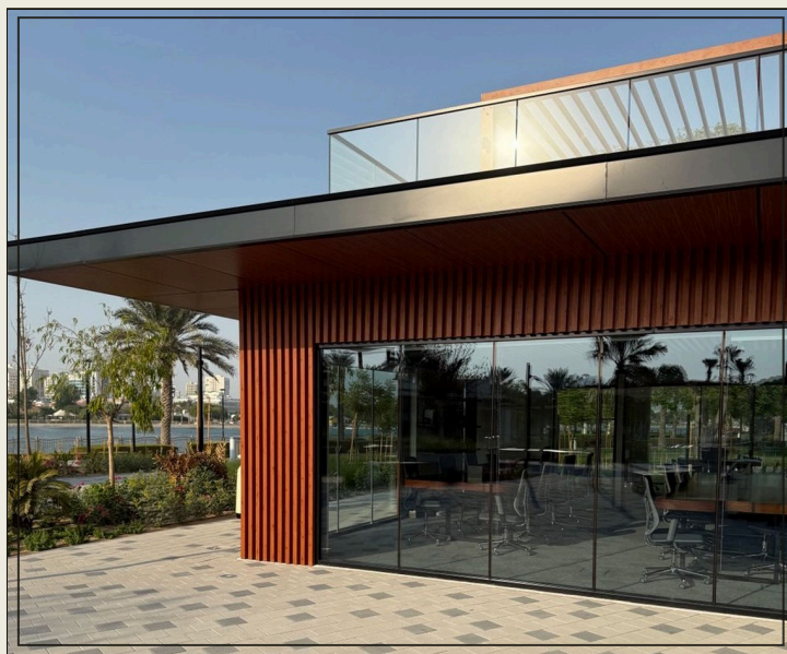
MODULAR, BY DESIGN. A factory-built pod meets the waterfront, its timber fins and glazing assembled on site.
